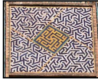
Figure 18: west Iwan, and square tiling that covered by Ali name.
